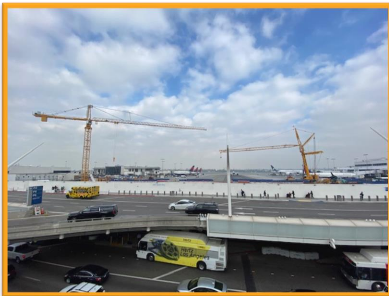
Airside cranes for Terminal 2 / 3 construction
