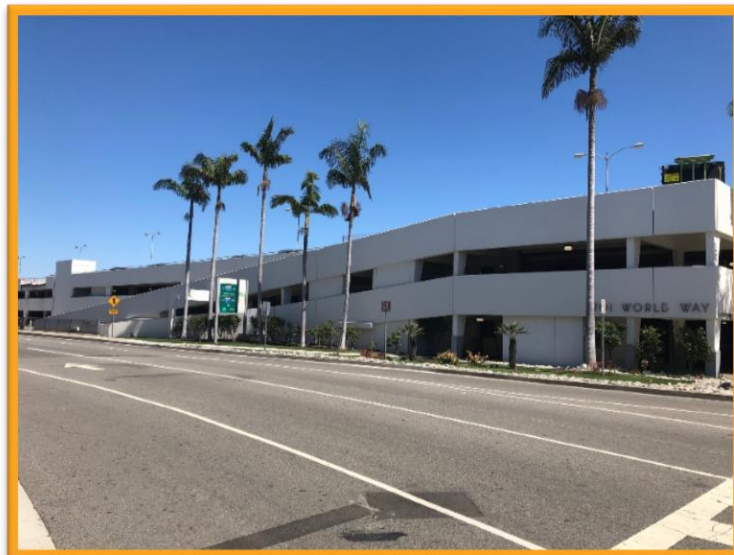
Parking Structure 7 Ramp Demolition
