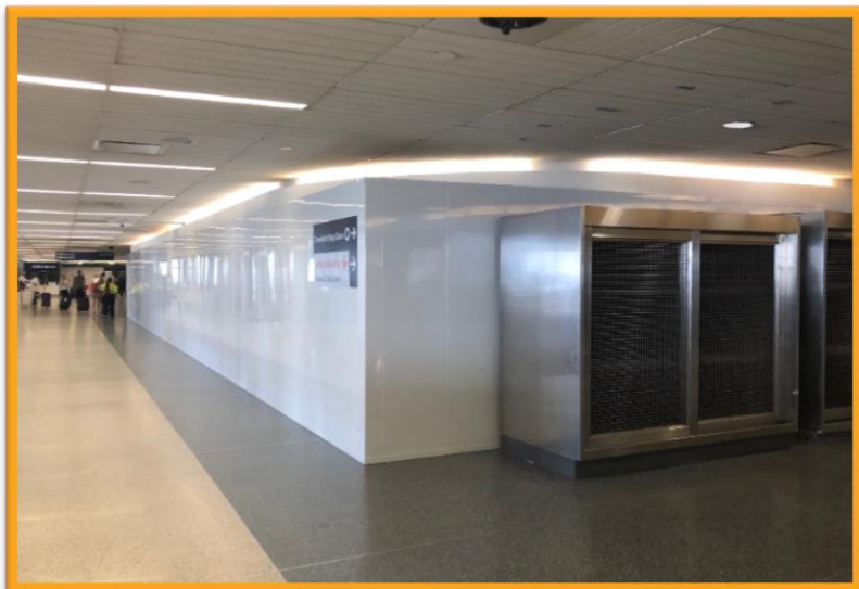
Terminal 6 Construction Barricades Bag Claim #1
