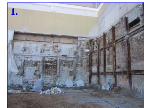
1. TBIT West Wall Demolition
