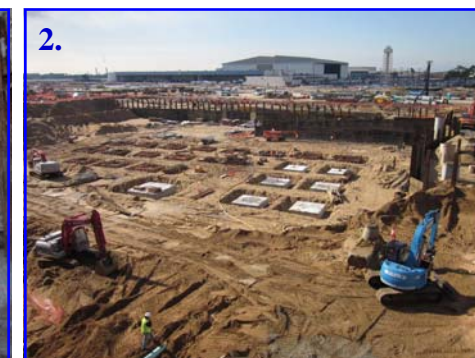
2. Core - Excavation & Foundations
