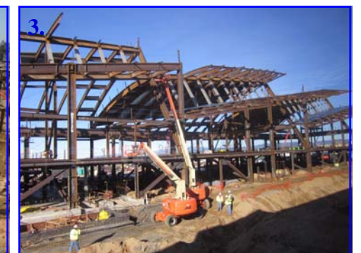
3. North Concourse Structural Steel
