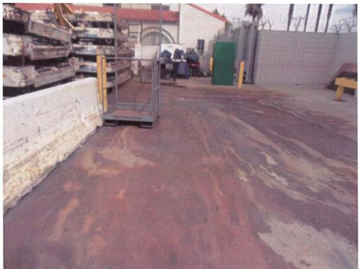
Photo 110: Acid or waste discharge resulted in the concrete pavement being stained and etched. There were no BMPs in place.
